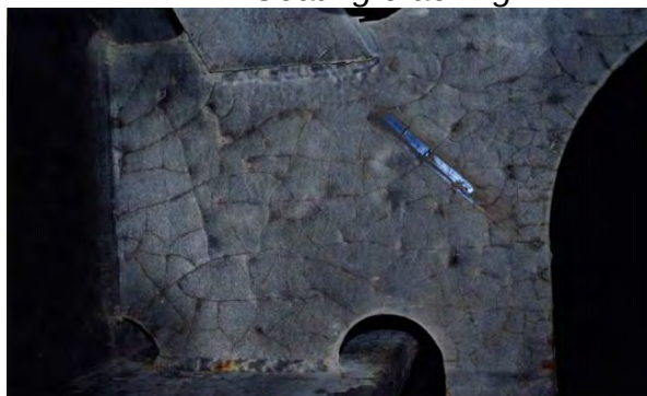
Coating cracking
