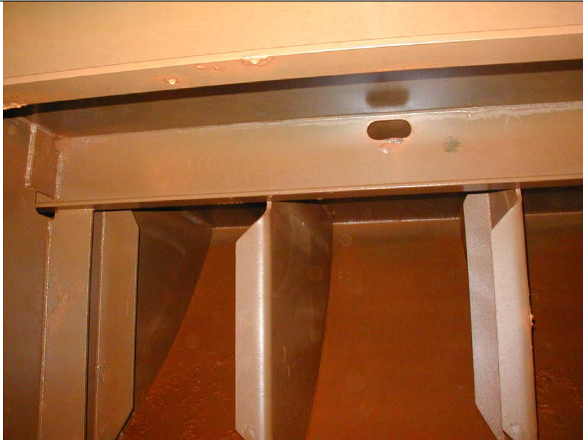
GOOD COATING CONDITION
